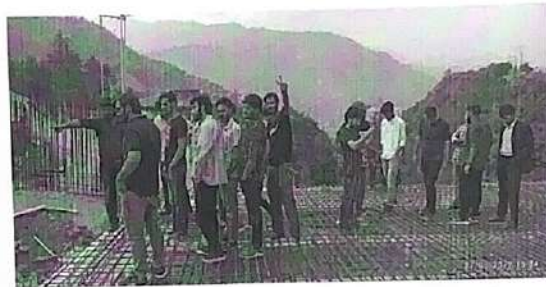
Students inspecting R/F of the Bridge Deck
